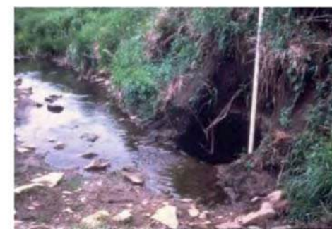
Karst conditions: Water wells in stream sinkhole. Photo Credit: Iowa DNR
